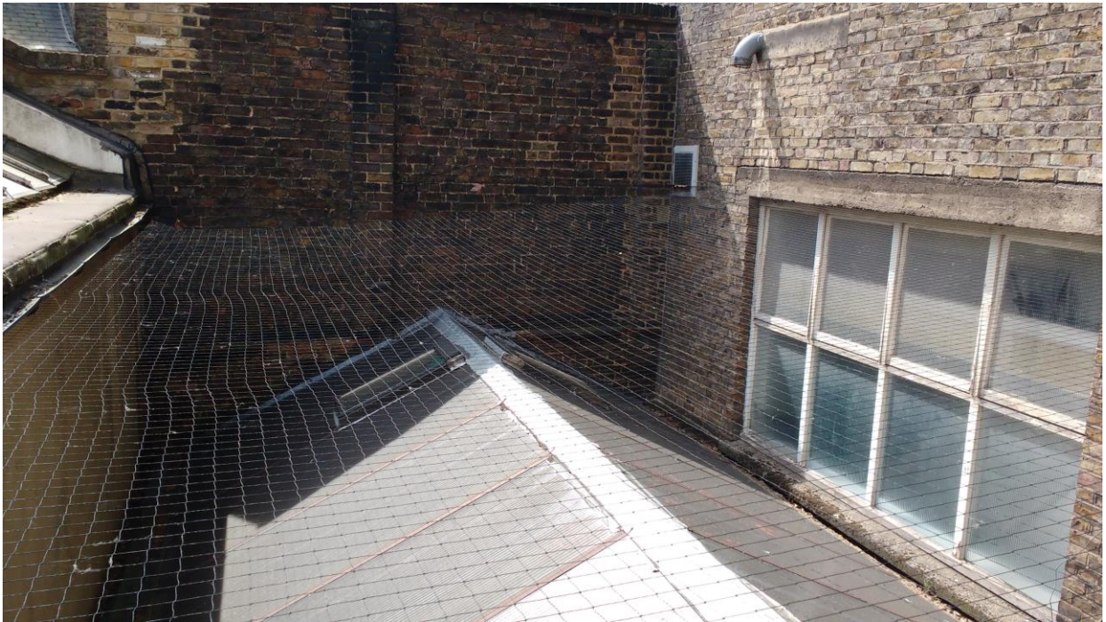
View of existing rear extension
